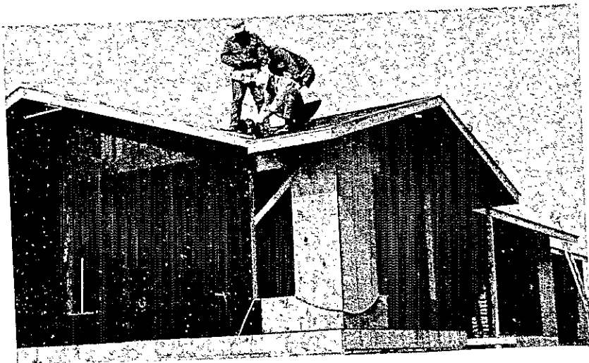
Residential Construction Program in action.
